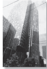
One of Amazon buildings in downtown Seattle
