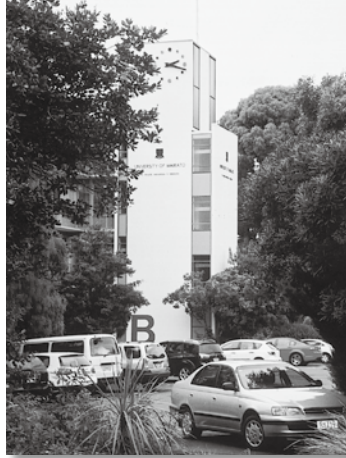
The University of Waikato Main Administration building
